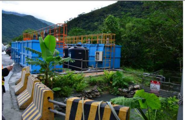
Photo 15: Mobile water treatment to treat water discharge from tunnel before discharging to river (To confirm effectiveness of water quality management, Koi fishes were put in the holding pond connecting to upstream collected water before discharging to river)
