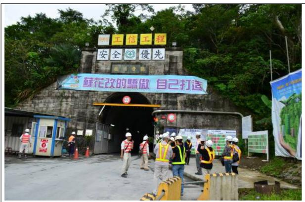
Photo 18: Overview of tunnel portal with traffic signalling control system and RFID positioning system of workmen and construction vehicles inside tunnel
