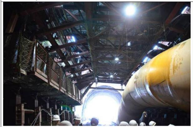
Photo 11 : Mobile steel frame formworks for tunnel lining construction  $% \left( 1\right) =\left( 1\right) \left( 1\right) \left($
